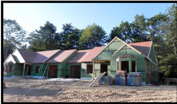
Duplex under construction at Wesley by the Sea
